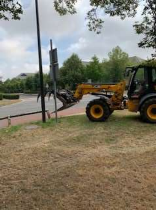
Bird's mouth fencing being removed.
